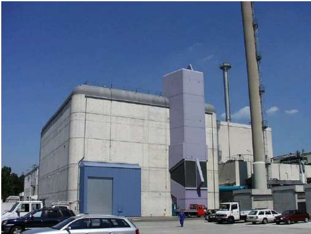
Fig. 4 External view of the vitrification facility (VEK).
