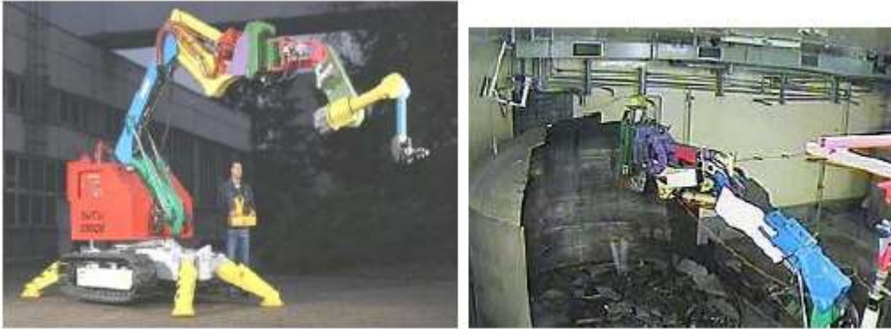
Fig. 7 (left) remote handled manipulator for various tools (right) storage tank demolishing
