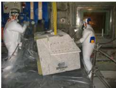
Fig. 6 Concrete block with pipe grommets.
